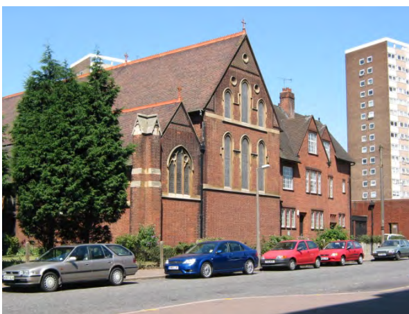
All Saints Church, Sutton Road ( outside of the SCAAP boundary )
