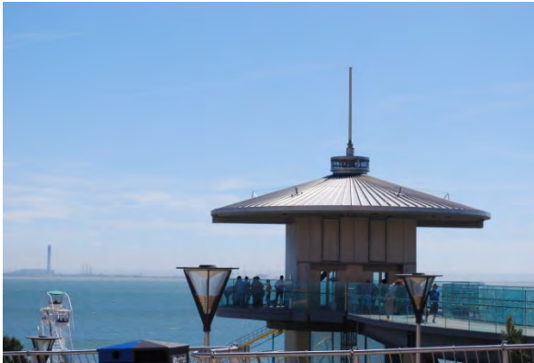
Pier Hill Observation Tower and Lift, Pier Hill (Central Seafront Policy Area)
